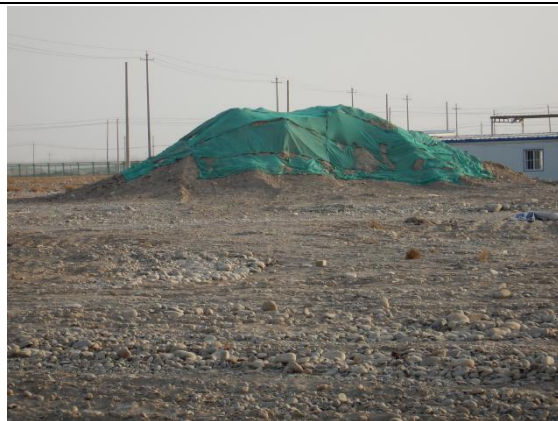
堆土临时苫盖
